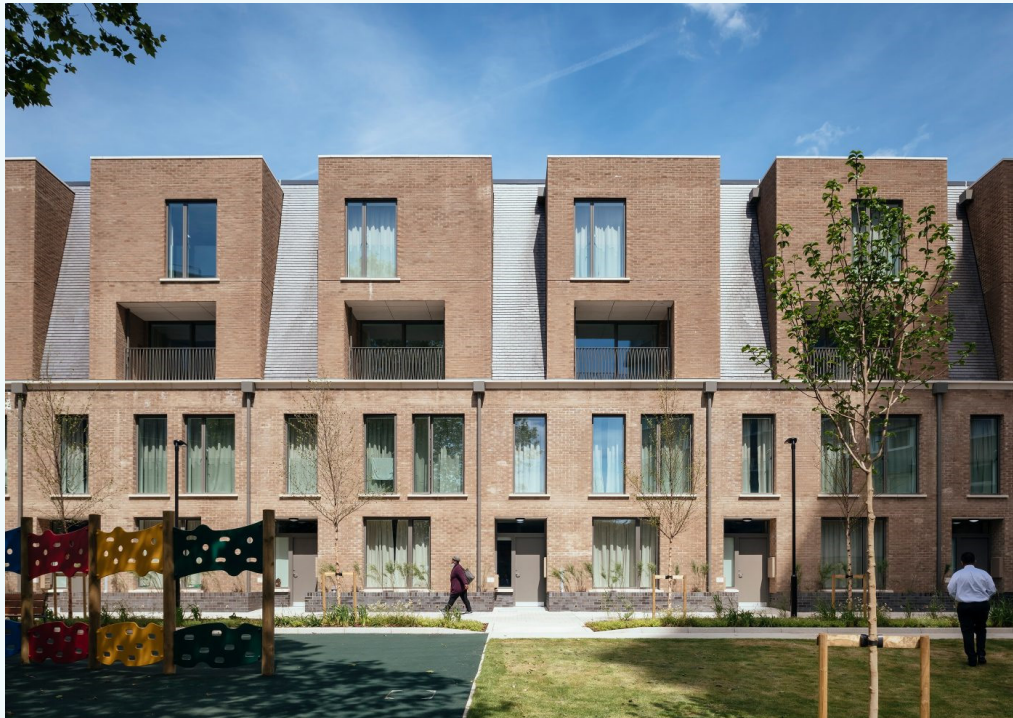
Agar Grove, Camden by Hawkins Brown is an example of a high quality residential development in an urban location which is Passivhaus accredited.
