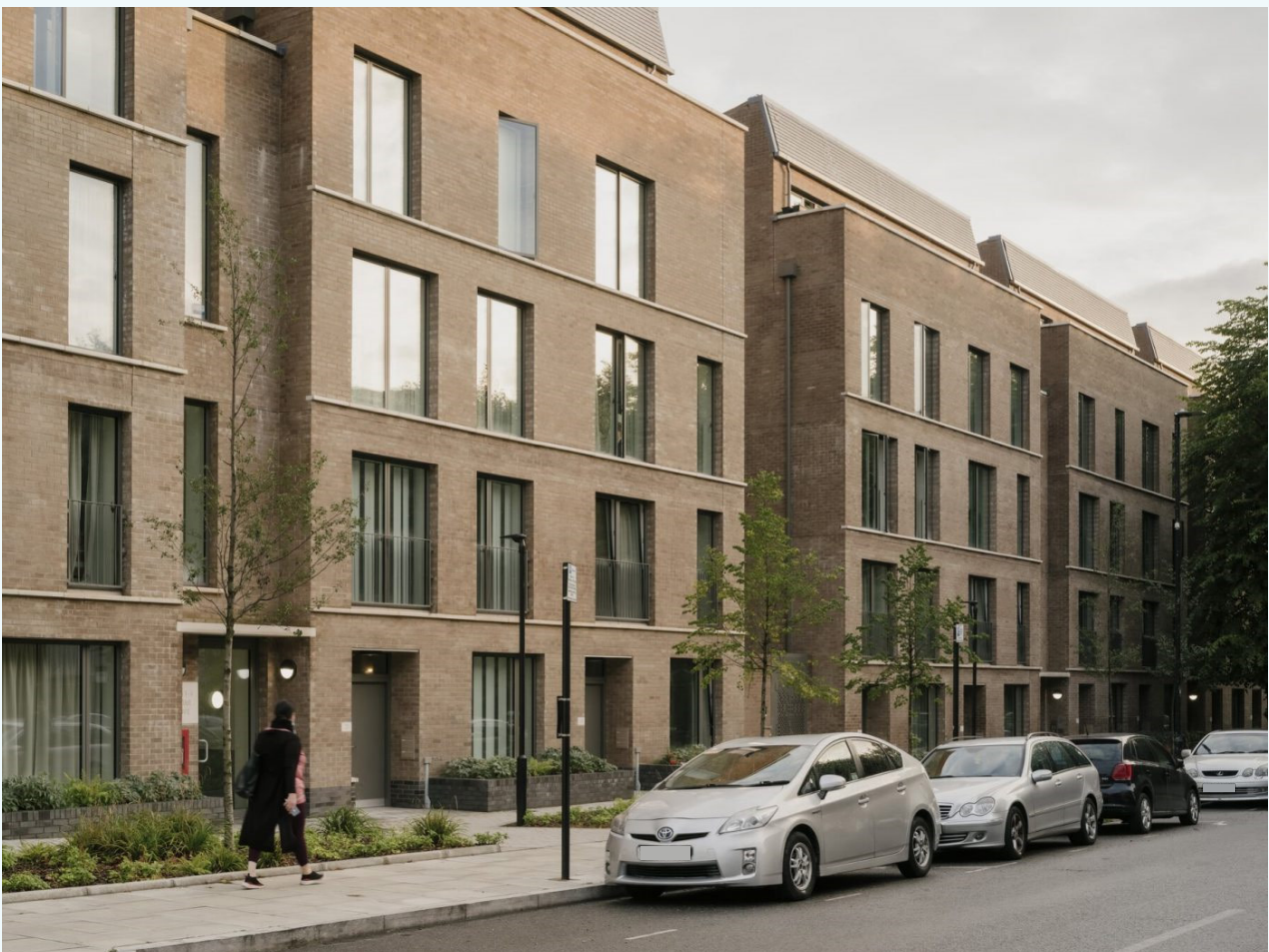
Sustainable design can often be invisible to passers-by. Agar Grove in Camden is an example of a contextually high development which is Passivhaus accredited and highly energy efficient.
